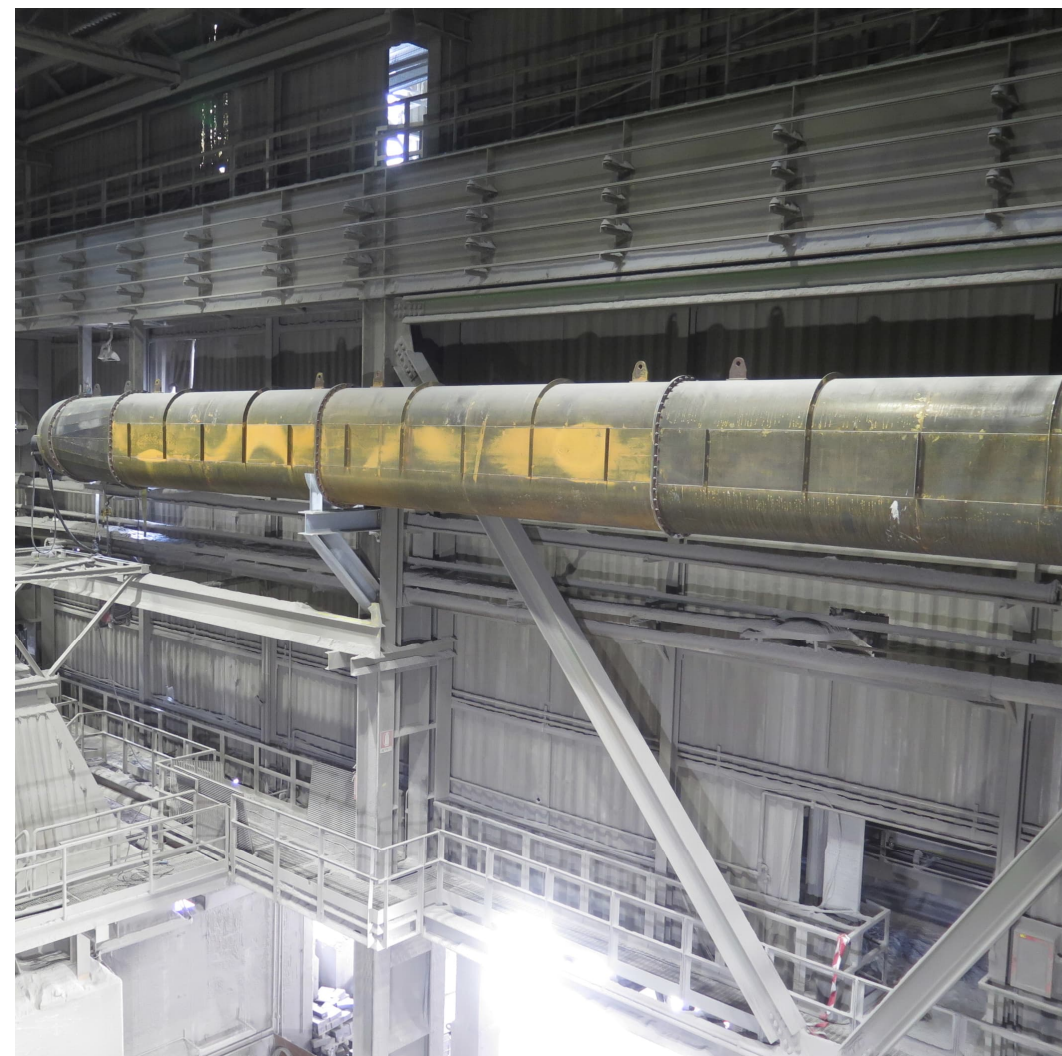
Obround shape to reduce print foot
