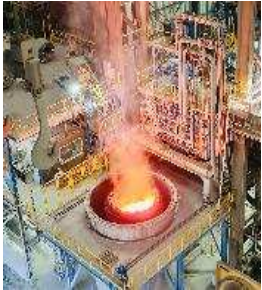
120 „short ton“ VD plant with mechanical pumps NUCOR Darlington, USA
