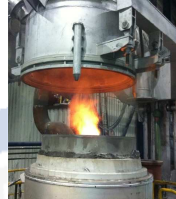
8t DETEM VD-VOD plant with mechanical pumps Lohmann, Germany
