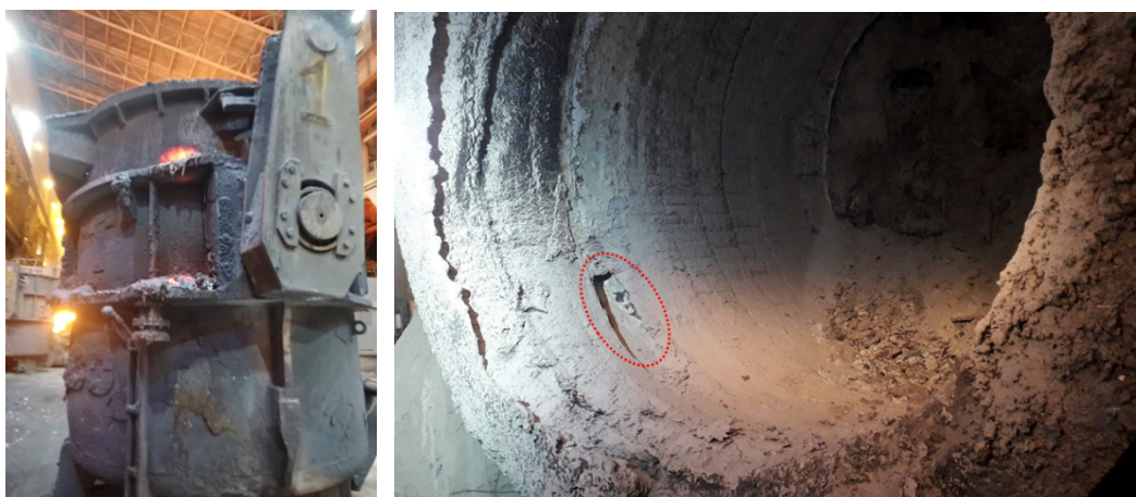
Figure 17. Refractory wear that caused hot spot on ladle shell during operation.
